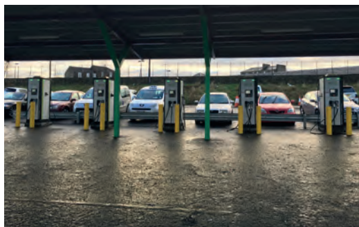
Left: Load distribution is essential for multiple charging stations with dual sockets
