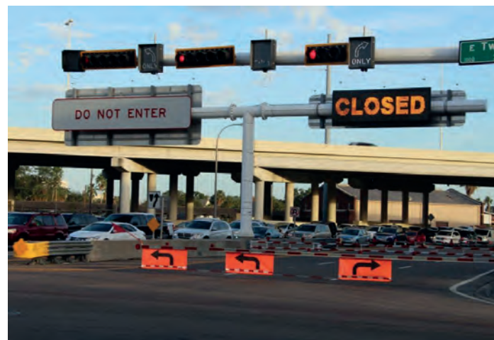
Above: The direction of flow on the reversible express lanes is changed depending on the time of day
