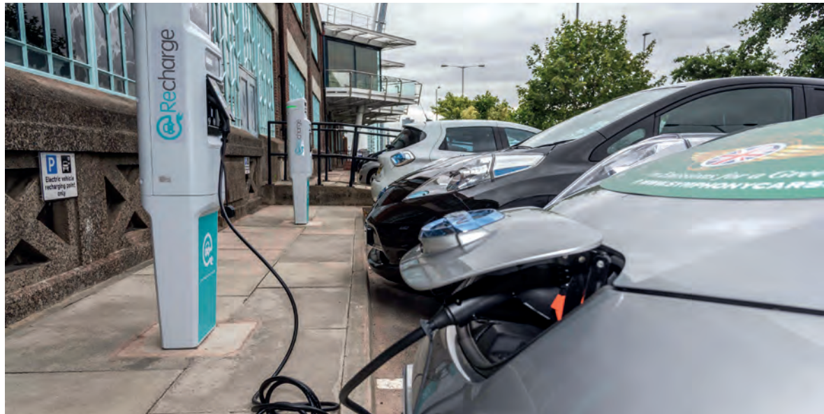
Left: Load distribution is essential for multiple charging stations with dual sockets
