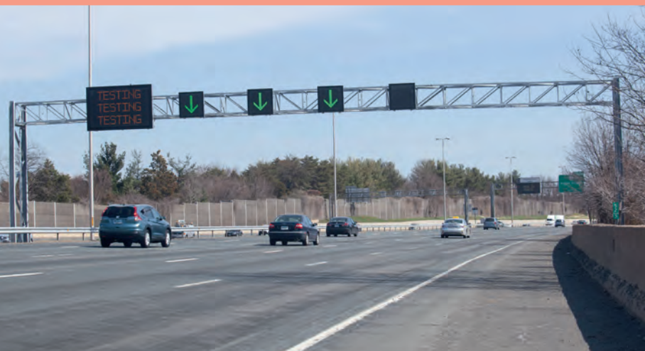
Left: The Virginia Connected Corridors, on I-66, US-50 and US-29, communicate information to vehicles using DSRC units (right) and VMS
