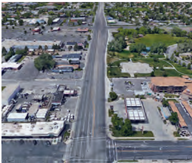
Above: An aerial view of Redwood Road, Salt Lake City, where UDOT has deployed connected vehicle technology on signals to help keep buses (opposite) running on time.
