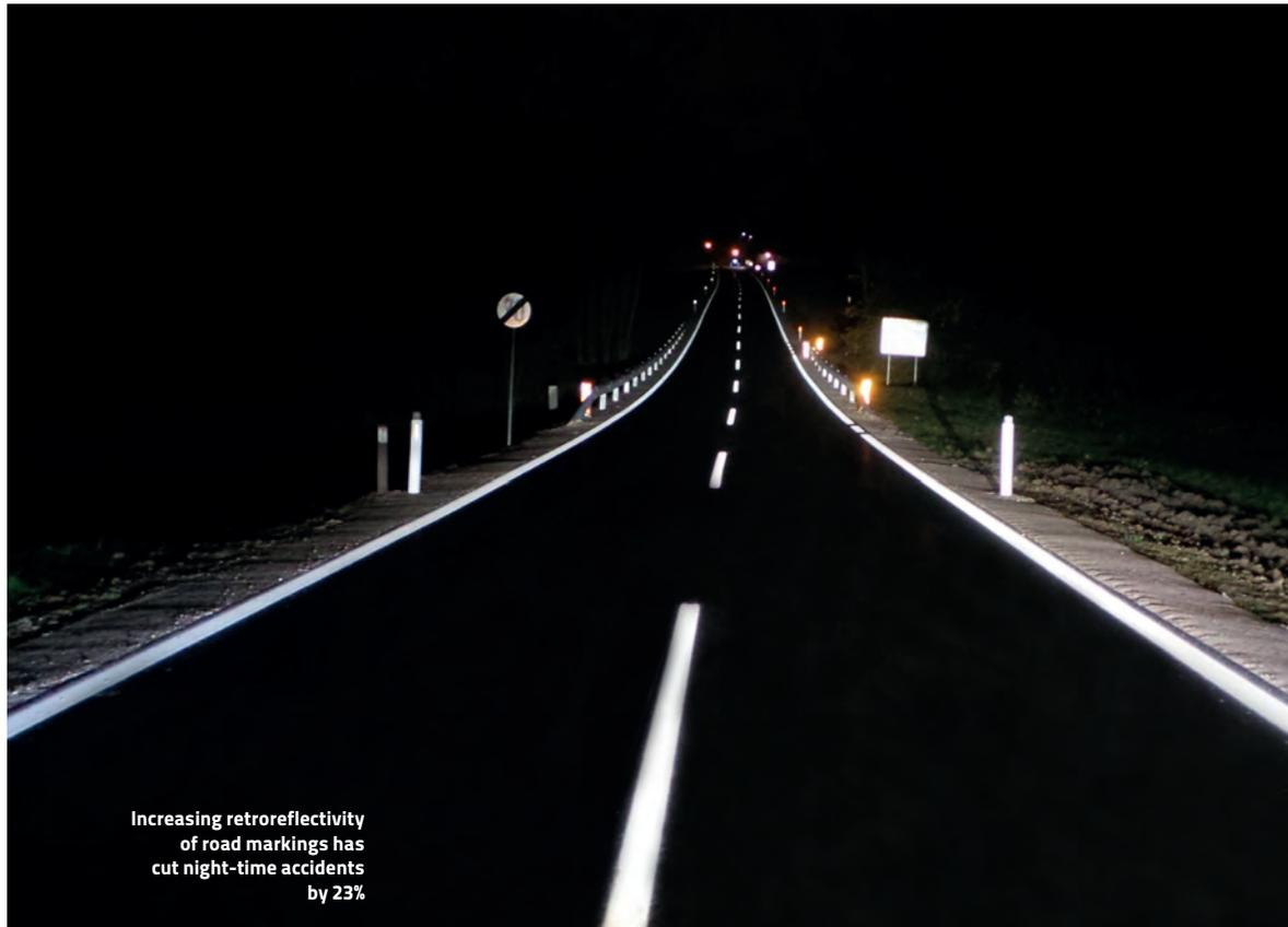
Increasing retroreflectivity of road markings has cut night-time accidents by 23%
