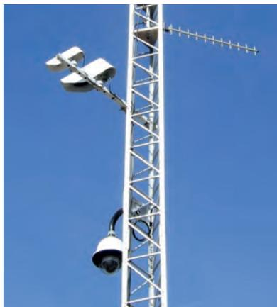
Left: A RWIS with Vaisala sensors installed in Snowmass Canyon on SH82 between Aspen and Glenwood Springs
